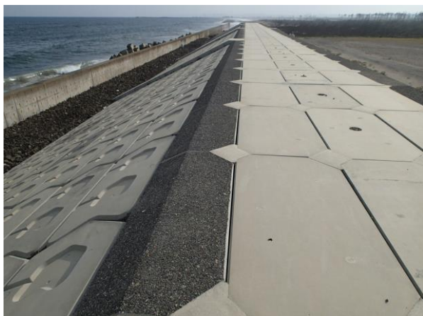
Fig. 2. Protection seawall by national recovery project (Sendai, Miyagi).
