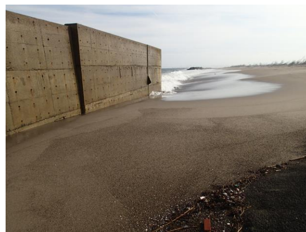
Fig. 1. Seawall basement (Sendai, Miyagi).
